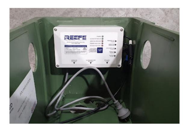
/A two-core monitor cable lead from the Control Panel is provided. The two-core monitor cable is to be connected to the terminal on the back of the house Warning Panel as illustrated below. Extension of the two-core monitor cable lead will be required.
